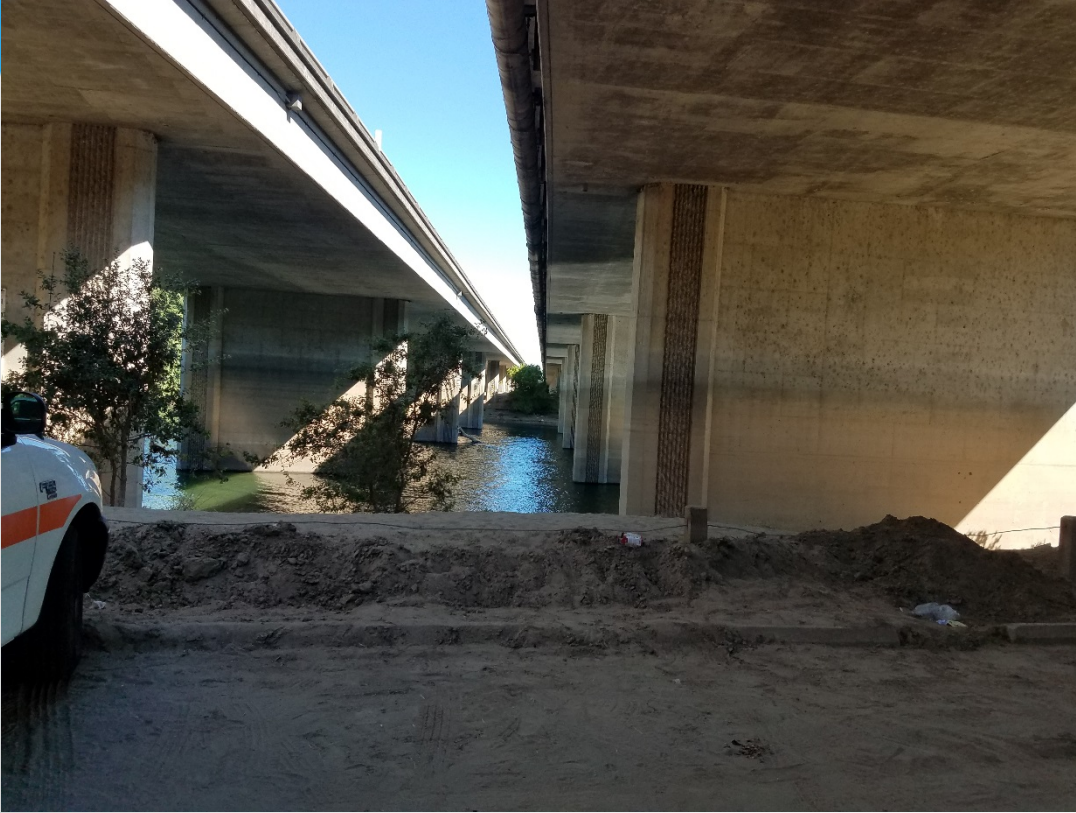
I-5 American River Bridge
