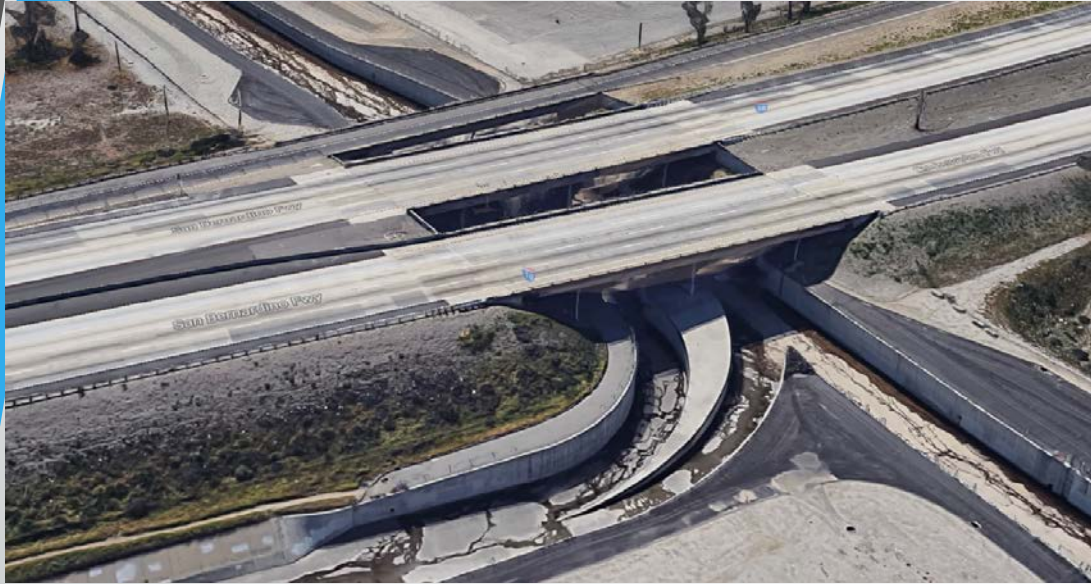
Rte. 10- Etiwanda- San Sevaine Flood Control Channel Bridge
