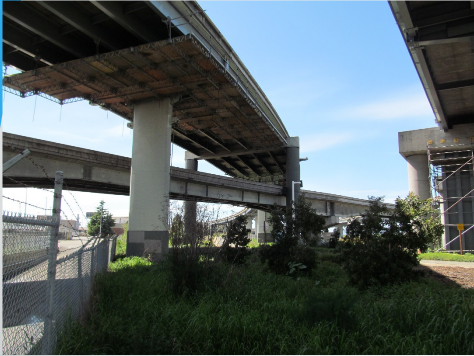
MacArthur Maze Interchange
