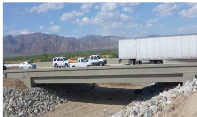
Figure 17. Interstate 10 Tex Wash Bridge after Replacement
