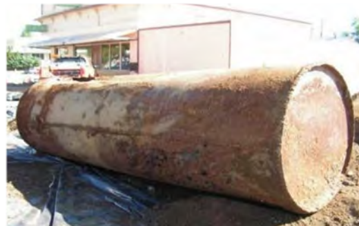
Underground Storage Tank Removed During a Remediation Project
