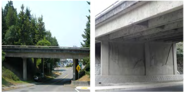
Figure 18. Trinidad Rd Undercrossing before and after Repair
