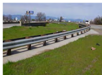
Figure 3. Vegetation control under guardrails reduce fire risks and pesticide use.
