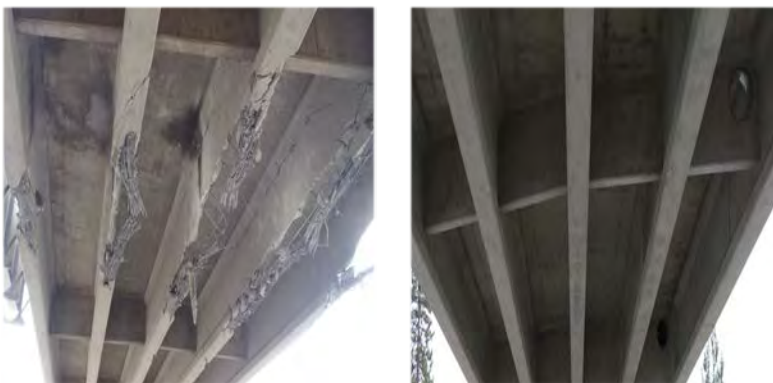
Figure 23. Walters Road Overcrossing before and after Repair
