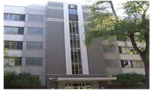
Figure 10. Caltrans Headquarters Built In 1936.
