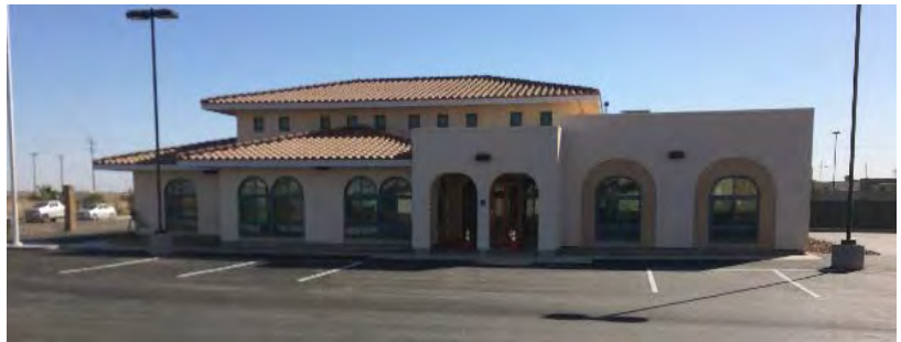
Figure 14. El Centro Maintenance Station and Equipment Sub-Shop after Relocation in 2016
