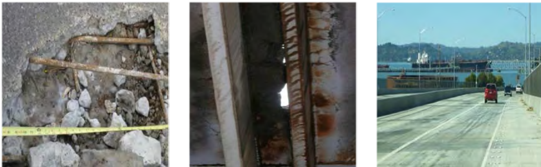
Figure 4. Scofield Ave Deck Spall Scofield Avenue Deck before and after Repair
