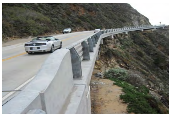
Figure 9. Permanent Restoration involved building a new viaduct.
