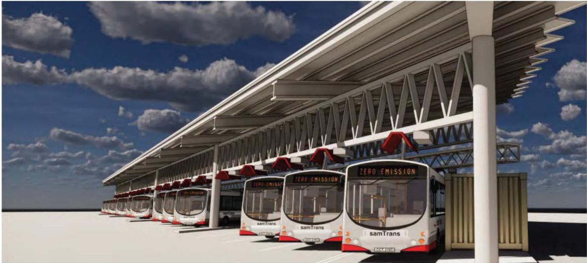
**Digital Rendering of Overhead Pantograph Charging Infrastructure**
