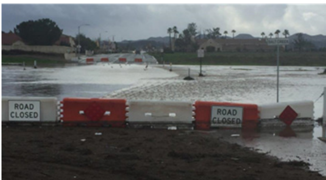
ABOVE: Recurring roadway closure during seasonal flooding
