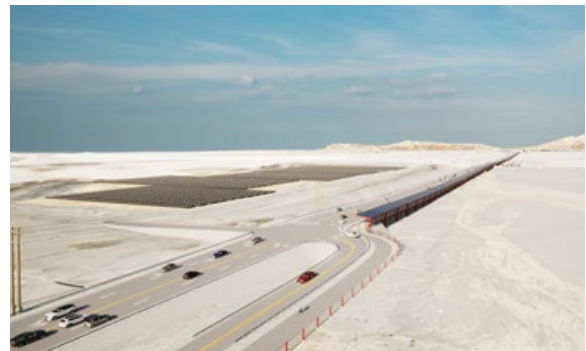
Sand mitigation fence to Amtrak's Palm Springs Station
