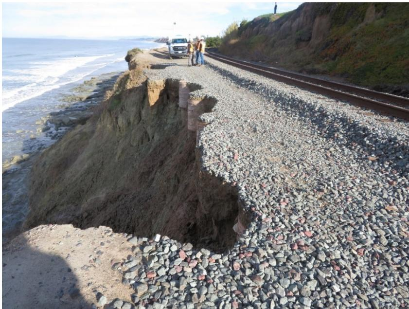
**Photo 3: Bluff Slide Thanksgiving 2019 Resulting from Surface Drainage over Bluffs.**
