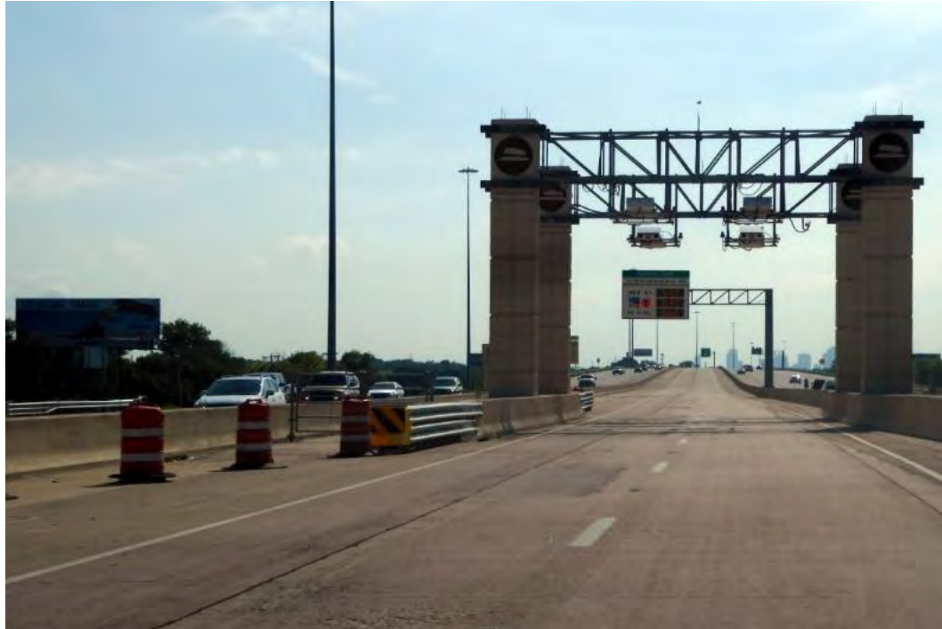
Figure 22: Example - Facility with Concrete Barrier
