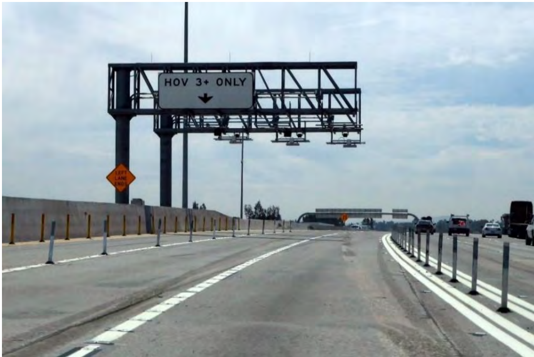
Figure 21: Example - Facility with Channelizers
