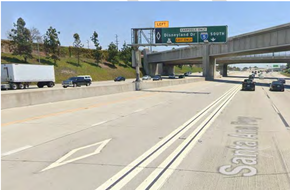
Figure 20: Example - Facility with Painted Buffer
