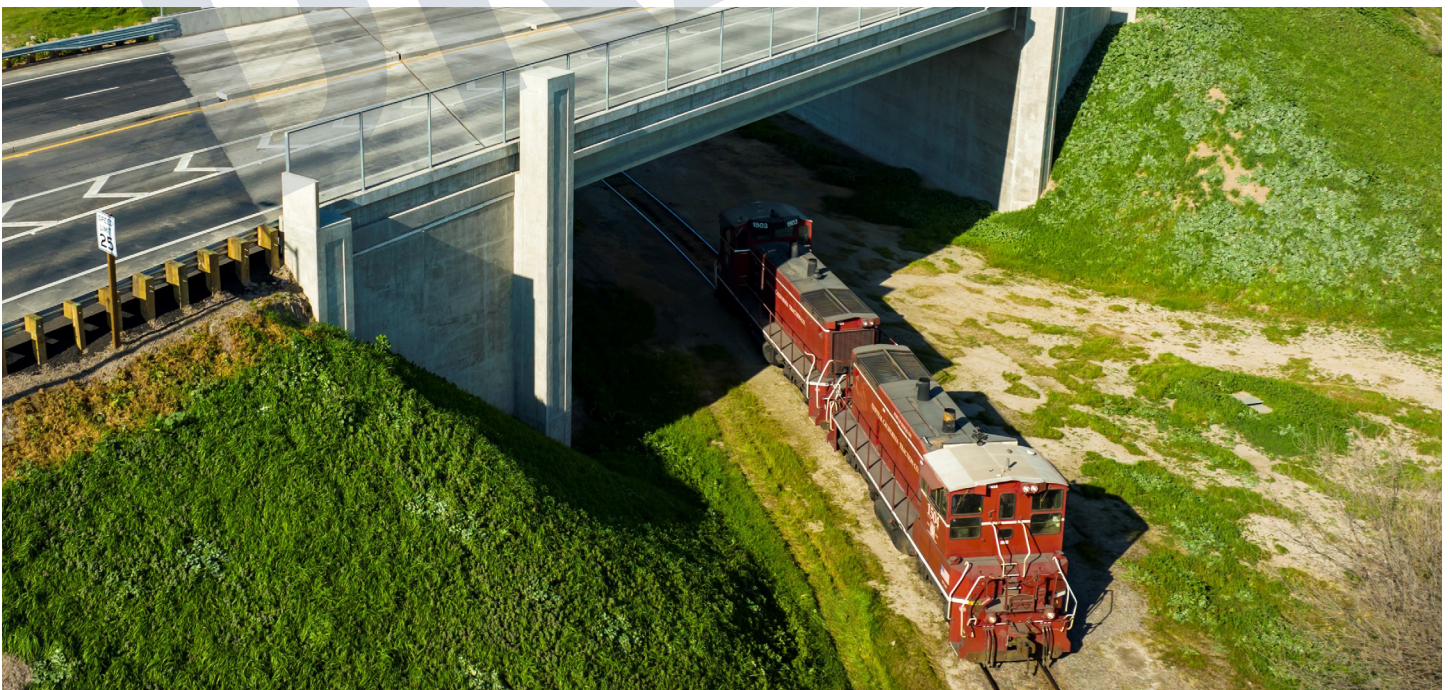
Funded through the Trade Corridor Enhancement Program, the Fyffe Avenue Grade Separation project constructed a four-lane overcrossing over the Fyffe Avenue rail line and removed an at-grade intersection. This project reduces travel times for vehicles entering the Port of Stockton, thereby facilitating the movement of goods. Removing the at-grade intersection also provides vehicle and rail safety improvements and enables a critical emergency evacuation route.
