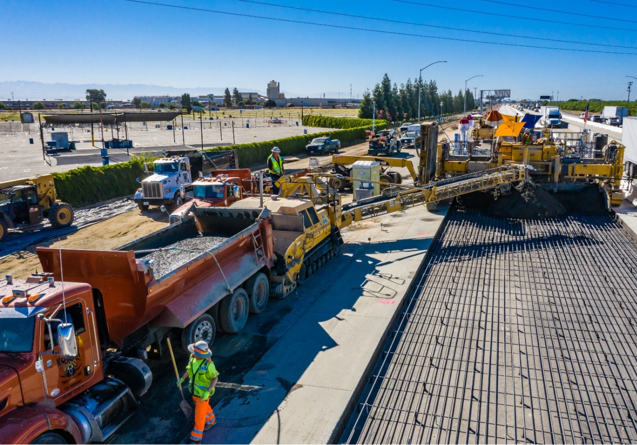
Route 99 concrete pavement- Fresno County from the City of Selma to Kingsburg
