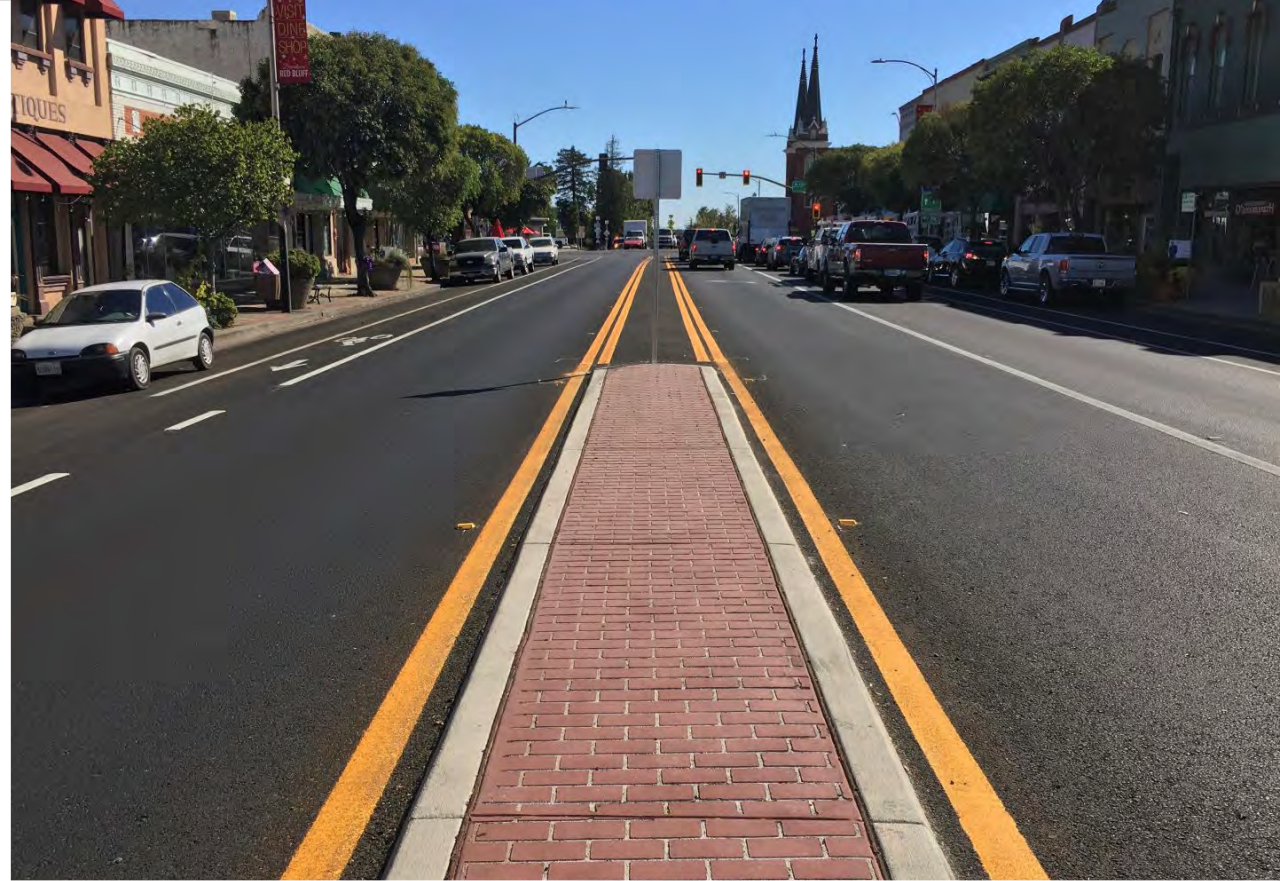
Pavement overlay with pedestrian/bike improvements – Red Bluff
