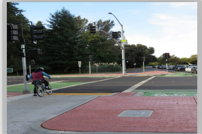
Curb Ramp/Signal Upgrades, City of Sacramento
