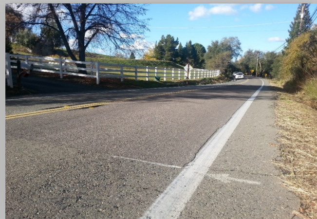
High Friction Surface Treatment, Placer County
