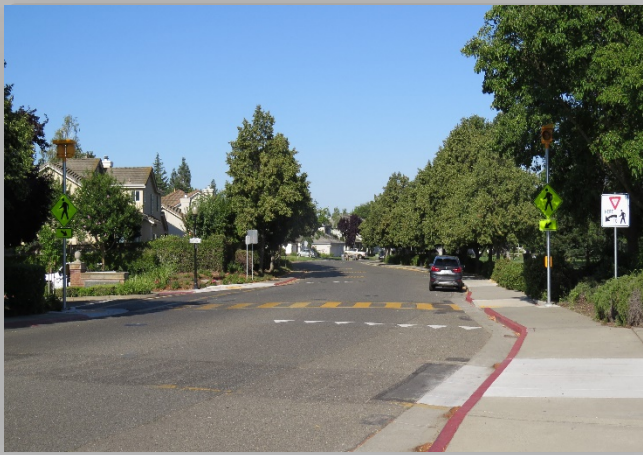
Ped Activated Beacon, Elk Grove
