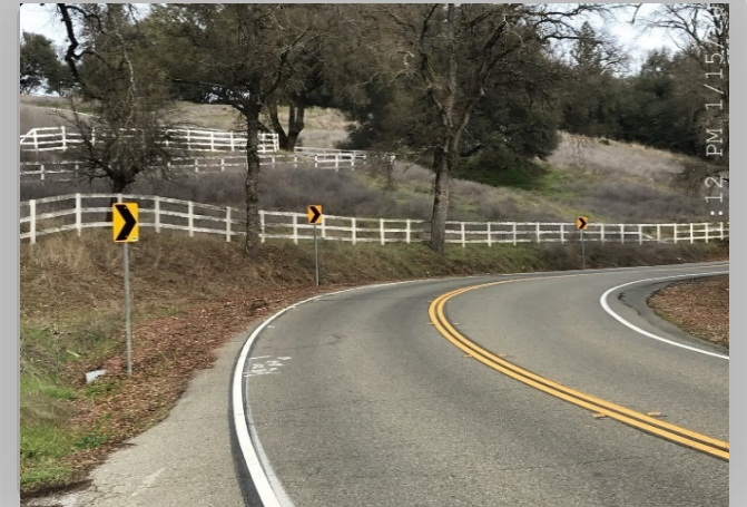
Curve Warning Signs, Nevada City
