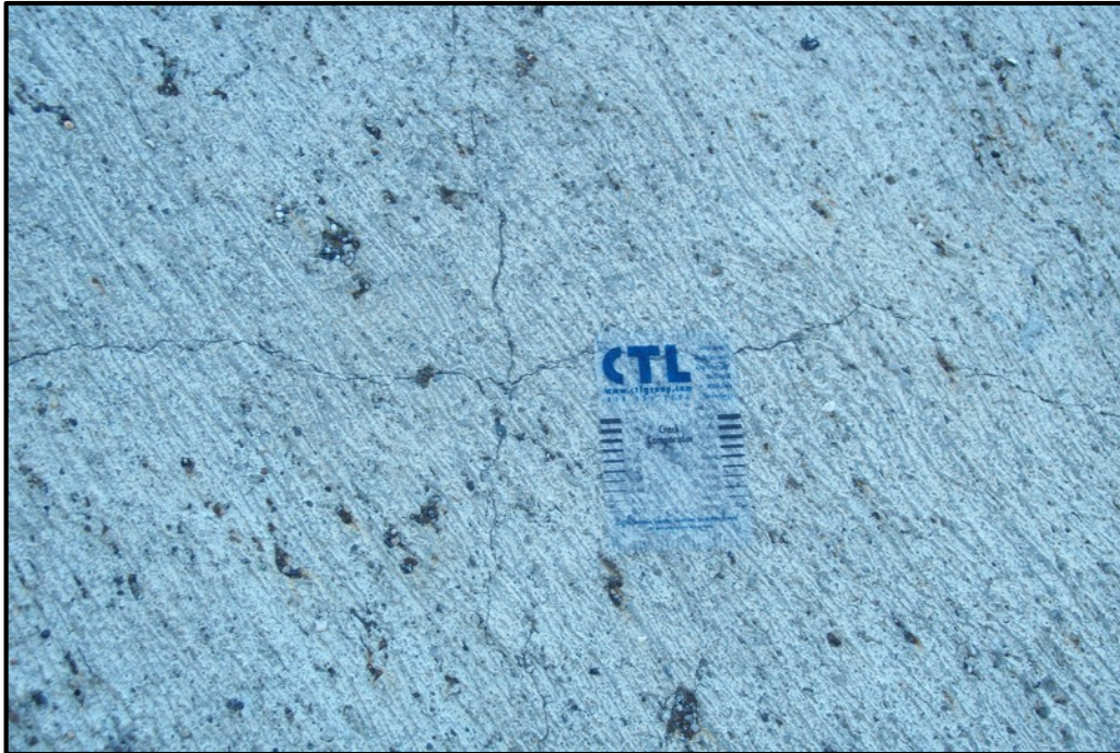
Close up of new bridge deck
