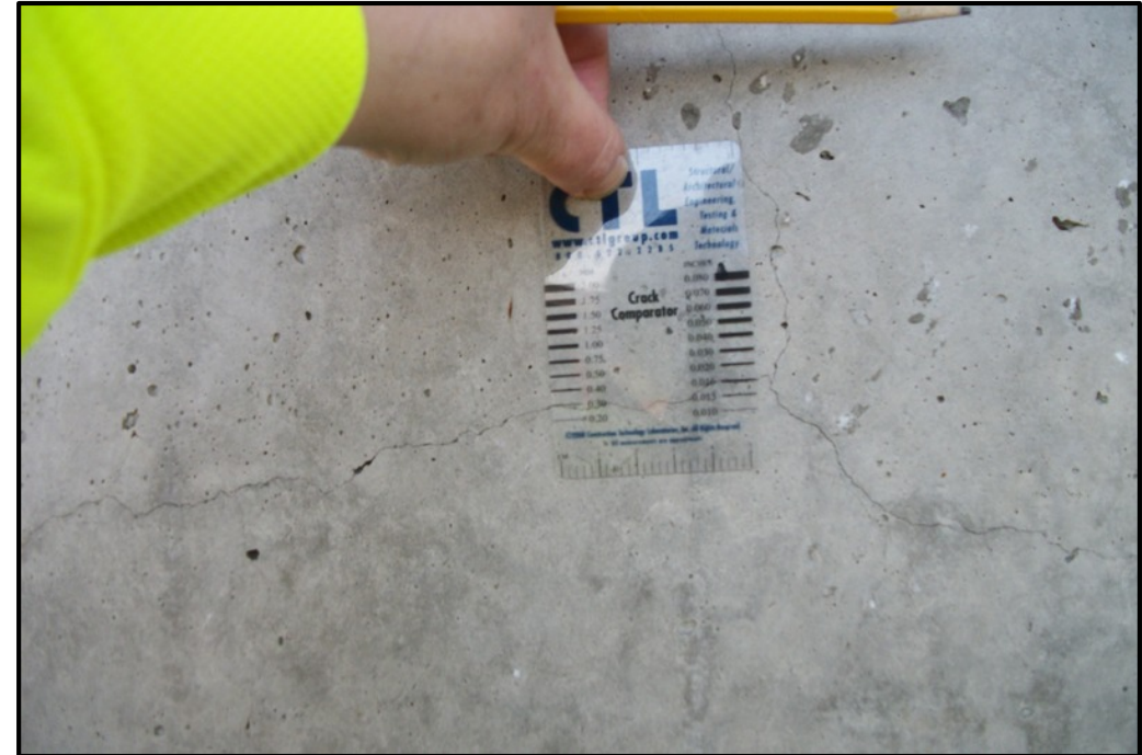
Close up of new bridge column
