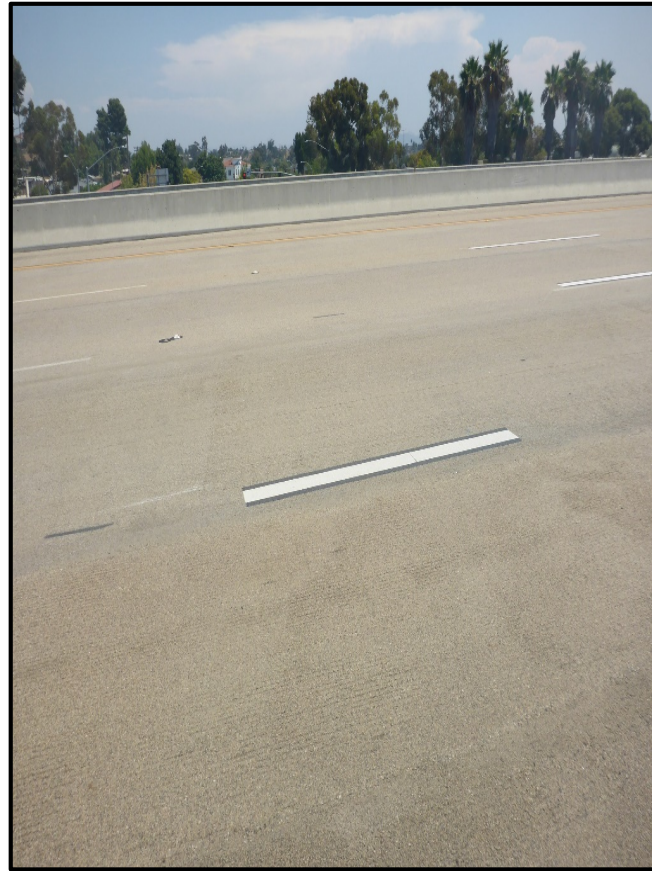
After – GOOD Condition Deck
