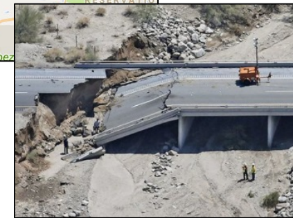
I-10 flooding & bridge collapse (July-Sept 2015)
