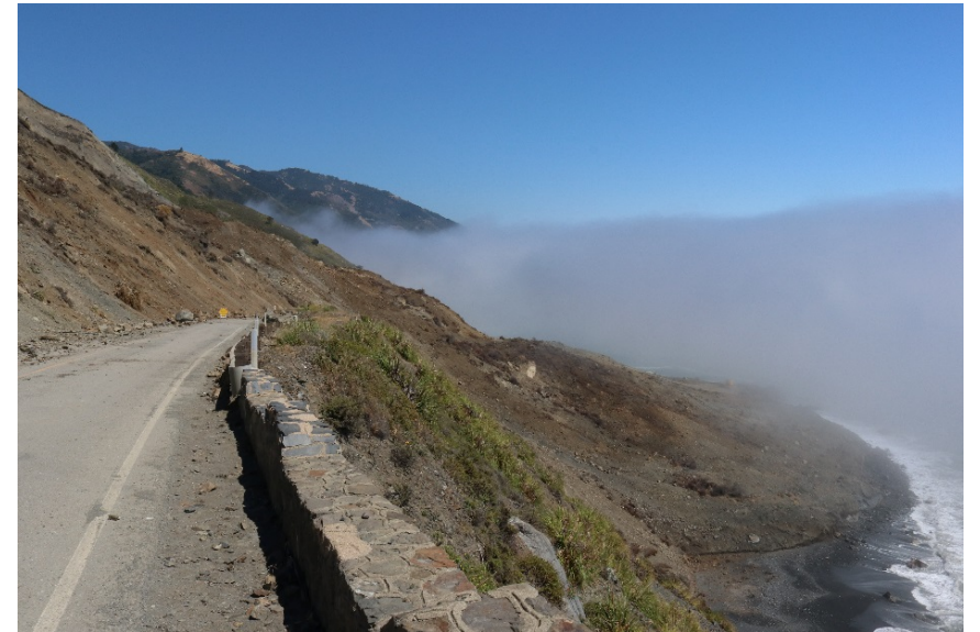
Highway 1, Mud Creek landslide, June 2017
