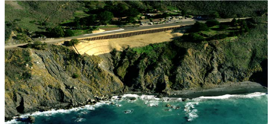
Rock slope protection along 101
